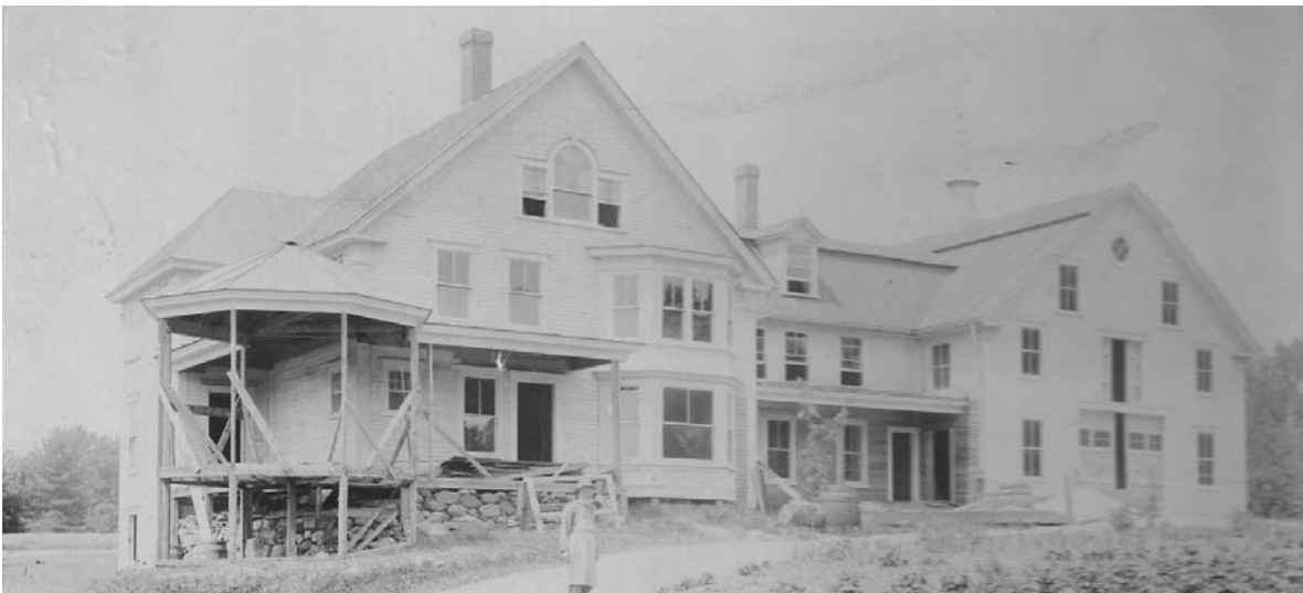
Building the new Gillis House in 1898 (now the Candlelite Inn)
