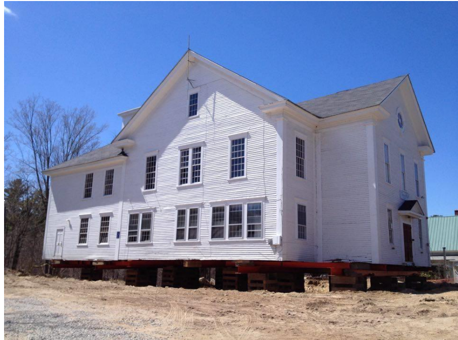
Lifted on steel beams and cribbing Photo by Maureen Brandon
