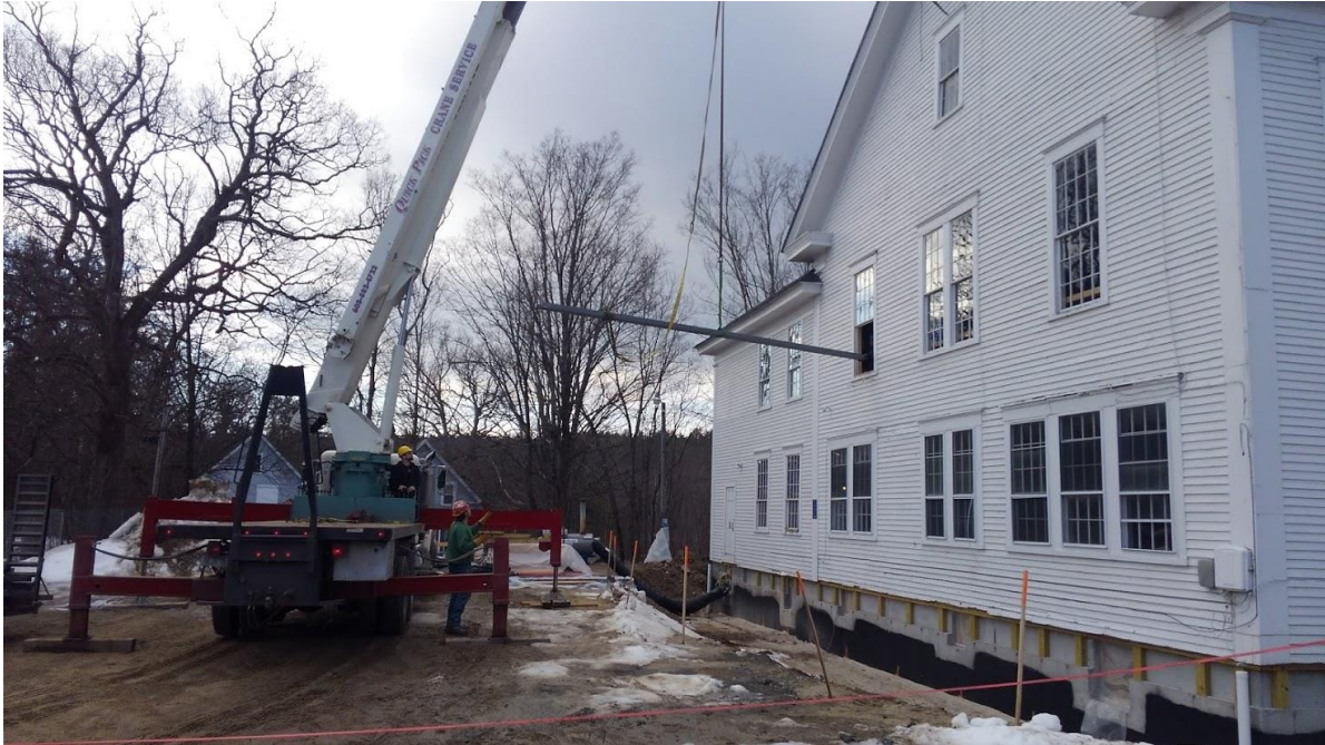
Steel to reinforce the stage being delivered Photo by Liam Ehrenzweig
