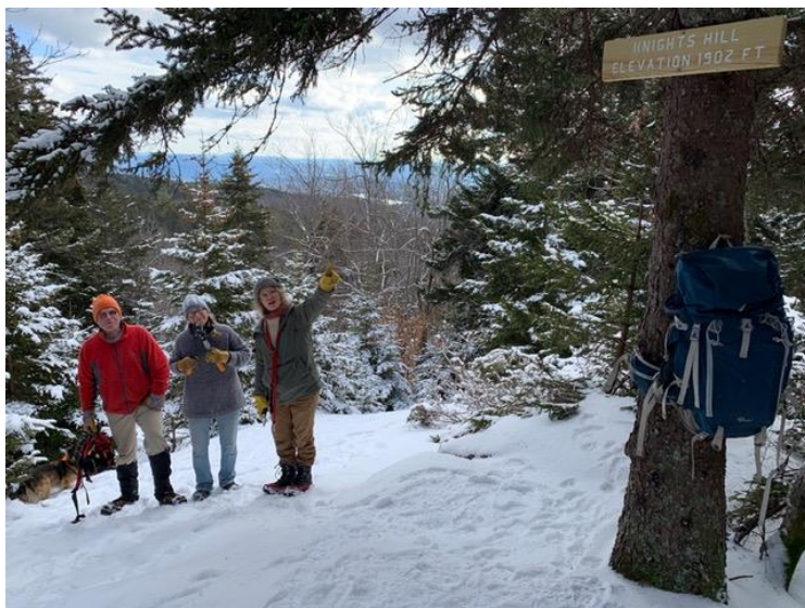
Knight's Hill Trail repair crew
