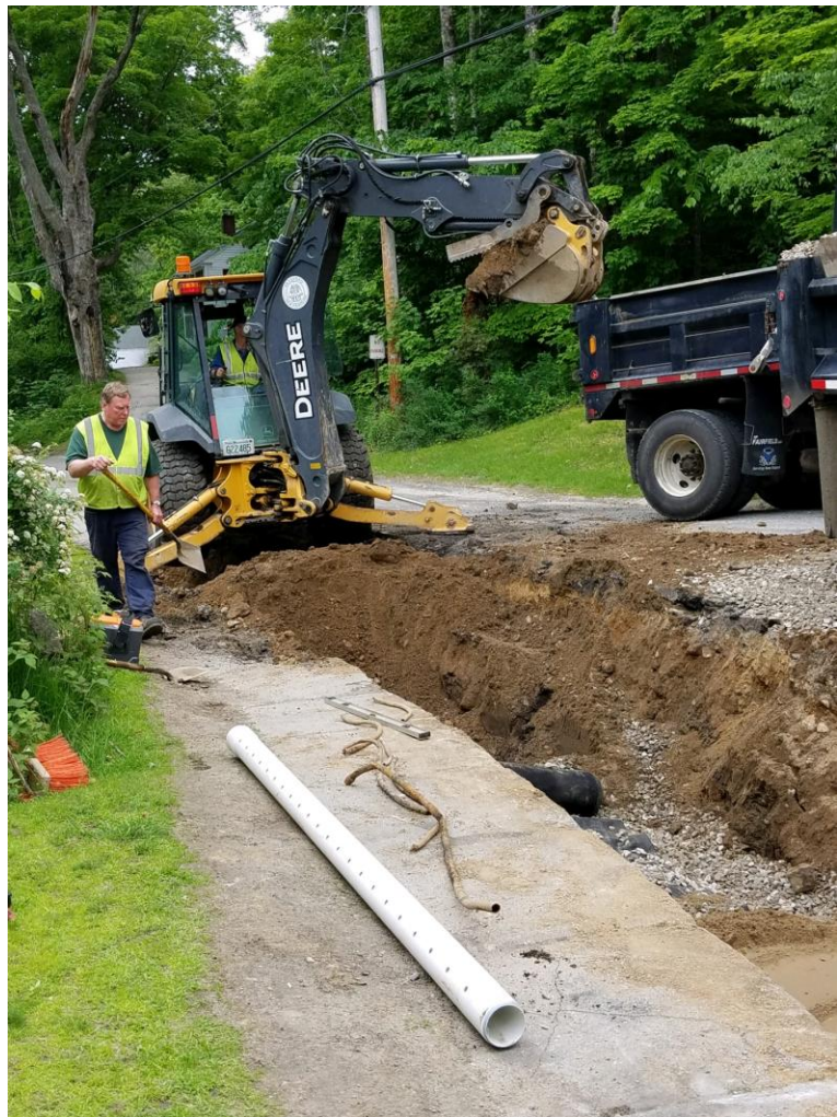
Highway Department Working on Water Street
