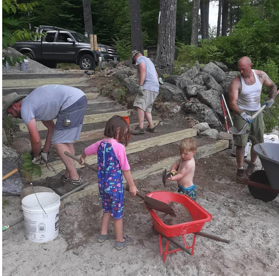
Rebuilding the French's Park Stairs Photo by Devin Pendleton
