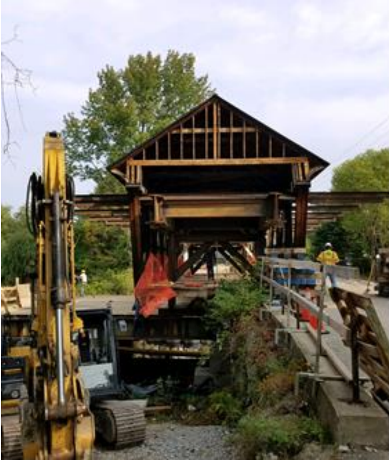
Bement Bridge being slid off its abutments Photo by Karen Hambleton
